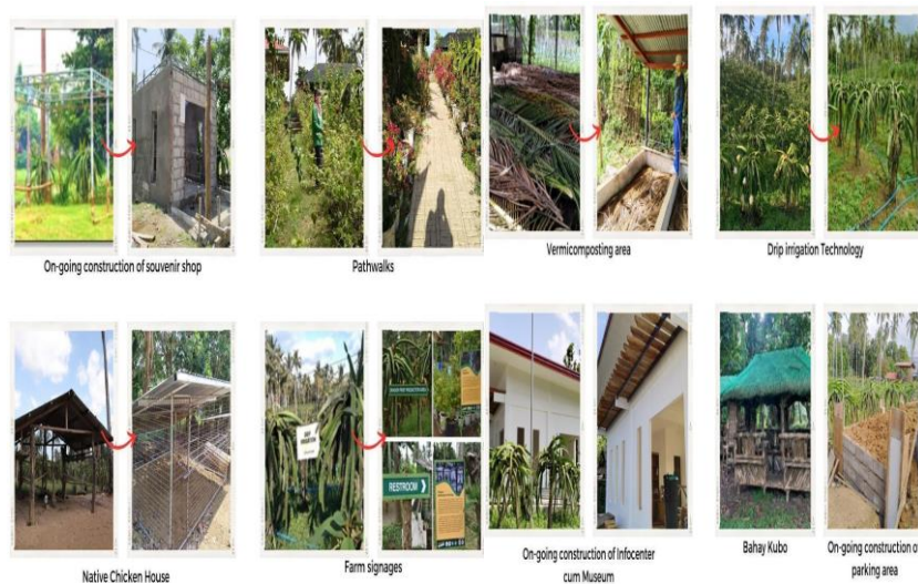
Figure 32. Improvement of some facilities in Silan's AgriFarm
